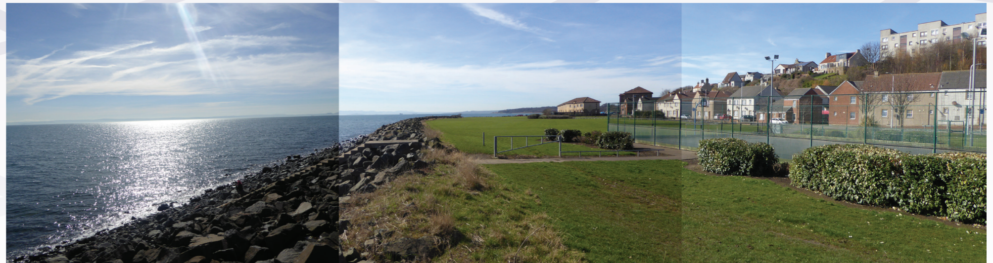
Before and after images of the Foreshore, showing improved cycle and foot access and grass mounds softening the impact of the rock armour
