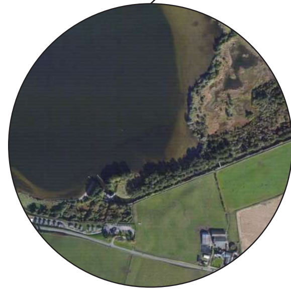
Site: Loch Leven sluice
