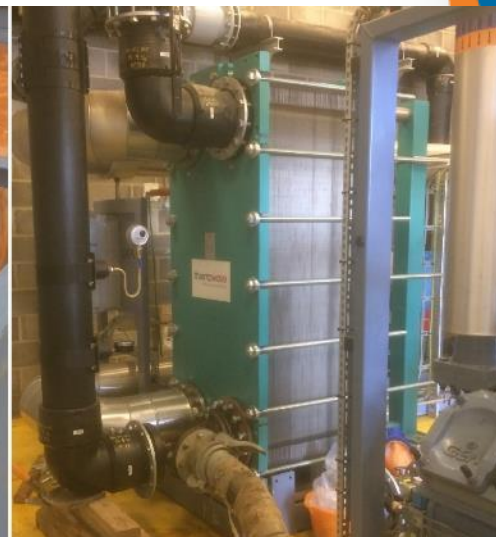
Circulating citric acid solution to remove ochre scaling from the plate heat exchanger at Abbotsford Road. Photo by © David Banks
