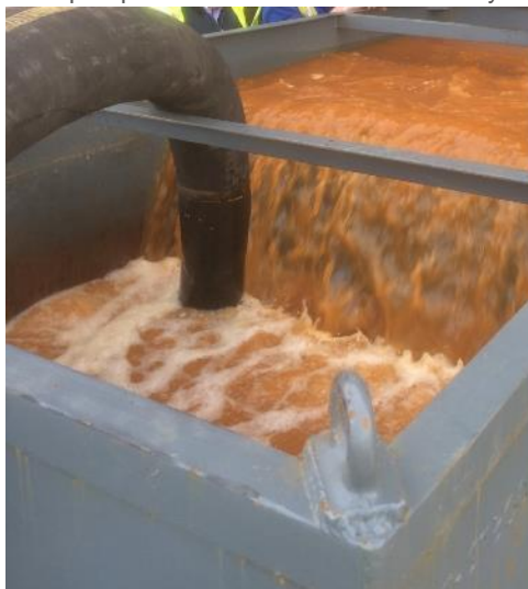
Circulating citric acid solution to remove ochre scaling from the plate heat exchanger at Abbotsford Road. Photo by © David Banks
